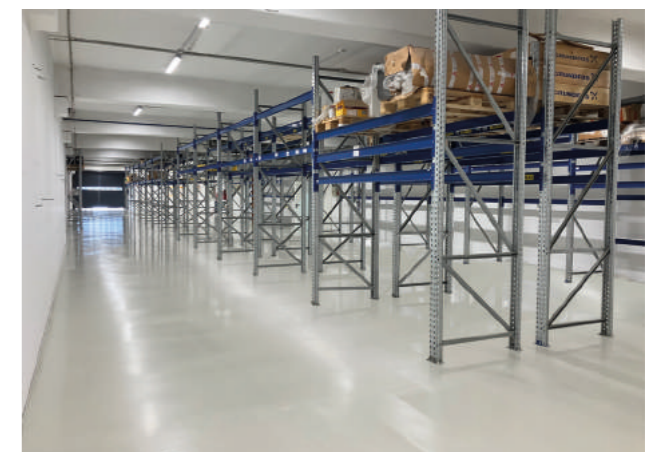
Low to medium duty warehouses and workshops
