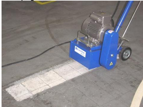
Scarifying concrete tiles
