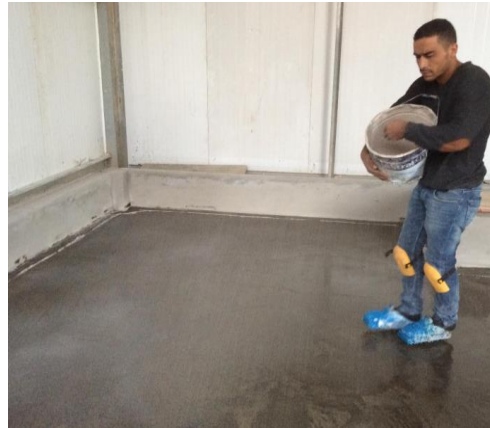
Broadcasting of the second layer of primer
