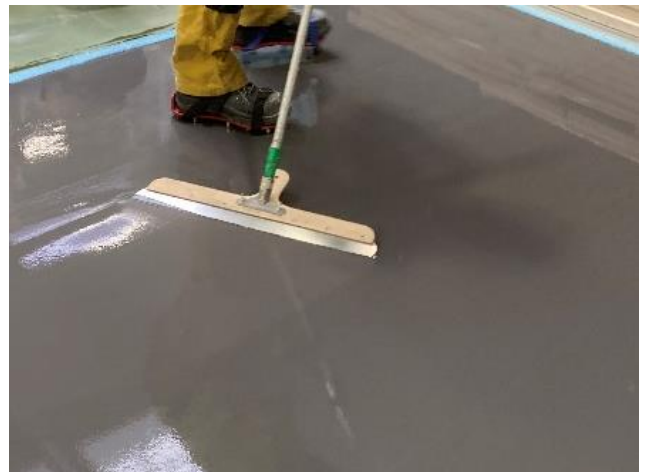
4. smoothing with surface blade
