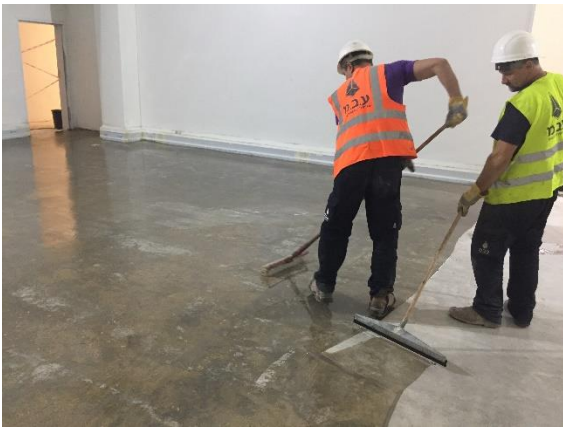
First priming layer application
