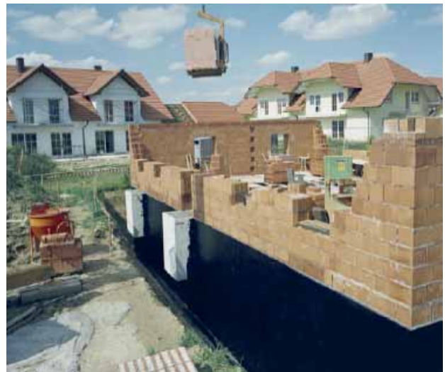
Tanking of an external basement wall with the thick bitumen coating PCI Barrapren.
