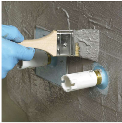
Fix PCI Pecitape 10 x 10 waterproofing collar and properly cover it with PCI Seccoral 2K Rapid.
