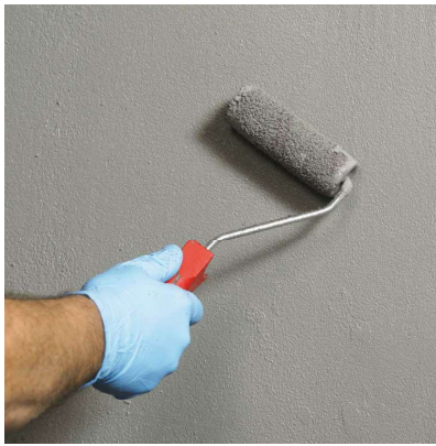
Apply first layer e.g. by roller or float covering the entire surface.
