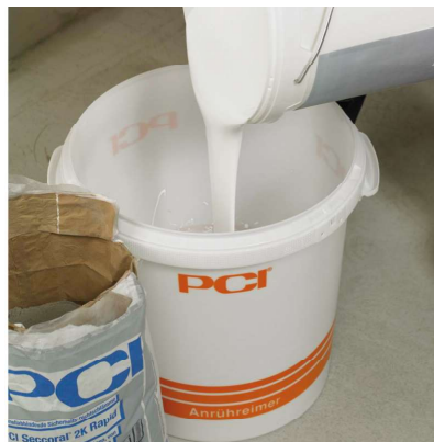
Pour liquid component of PCI Seccoral 2K Rapid in a clean container.
