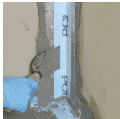
Install PCI Pecitape waterproofing tape in corners.
