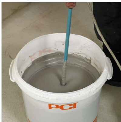
Mix PCI Seccoral 2K Rapid to a homogeneous compound for the application by trowel (1 a).
